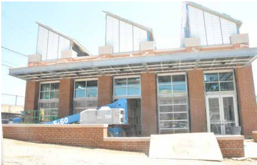
New Dance Place building under construction
