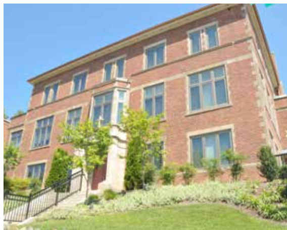
St. Martin's Convent Building
