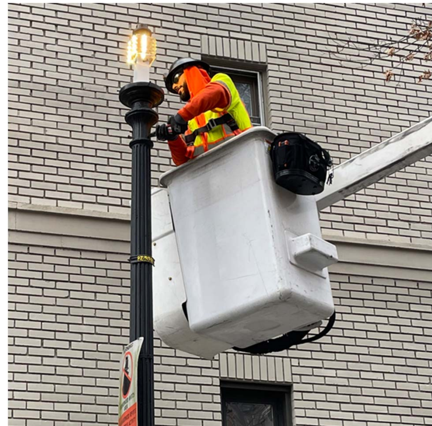
LED streetlight installation
