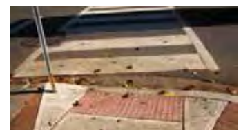
CURB RAMP WITH ADA TACTILE WARNING TILES
