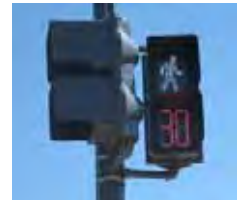
TYPICAL COUNT DOWN PEDESTRIAN SIGNAL
