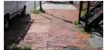
COMMON BRICK SIDEWALK DETERIORATION
