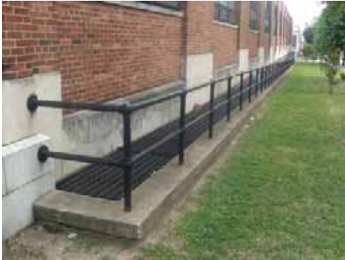
Areaways are used to get light into lower levels of commercial or industrial buildings.
