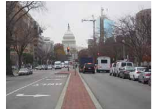
Medians that are less than 4 feet wide must be a hardscape material like stamped concrete, brick, flagstone, or exposed aggregate concrete.
