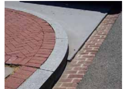
The standard curb radius for all driveways is 6 feet.
