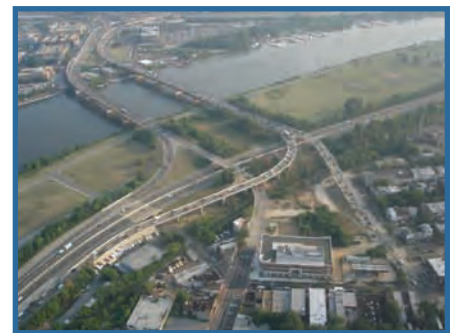
The existing 11th Street Bridges
