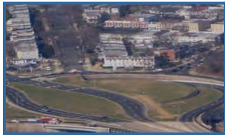
Barney Circle existing conditions
