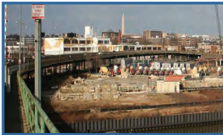
Douglass Bridge conditions prior to construction
