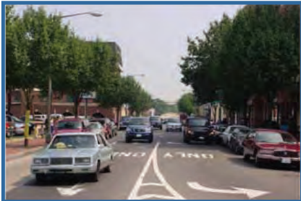
Martin Luther King, Jr. Avenue prior to reconstruction.
