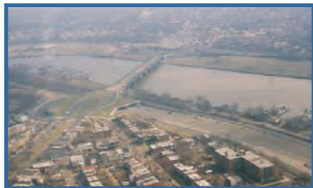
Southeast Boulevard existing conditions
