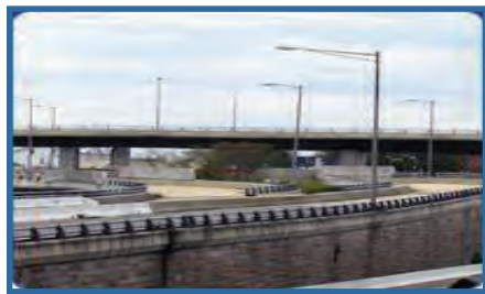
11th Street Bridge Existing Conditions
