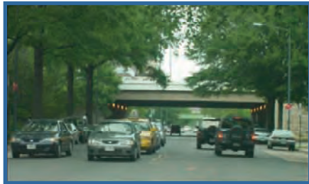
4th Street SW Existing Conditions
