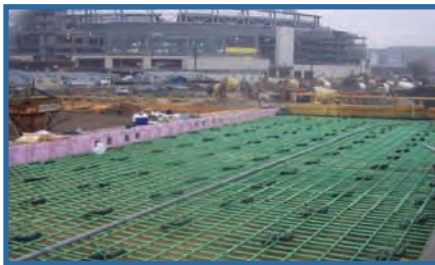
Douglass Bridge construction work, August 2007
