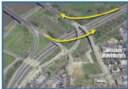
Movements missing from the existing 11th Street Bridges configuration
