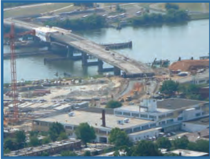
The Frederick Douglass Bridge undergoing renovations in 2007
