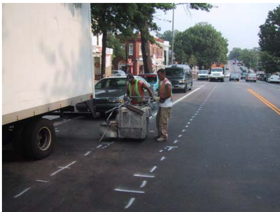
DDOT street maintenance crew applies thermoplastic bike lanes.
