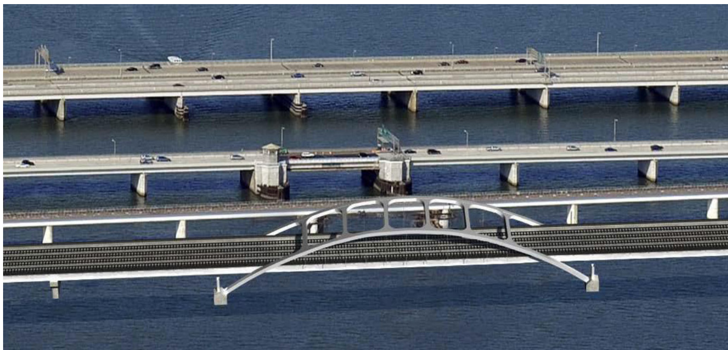
Image 9.4: Steel Tied Arch Bridge
