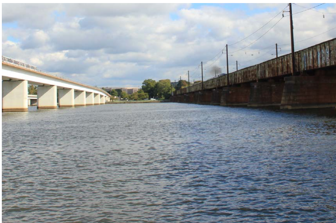
Image 8.2: District Shoreline between the Long Bridge and Metrorail Bridge
