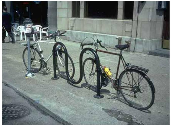
Examples of bicycle racks that are not approved. The designs do not properly support bicycles and lead to improper and inefficient parking.
