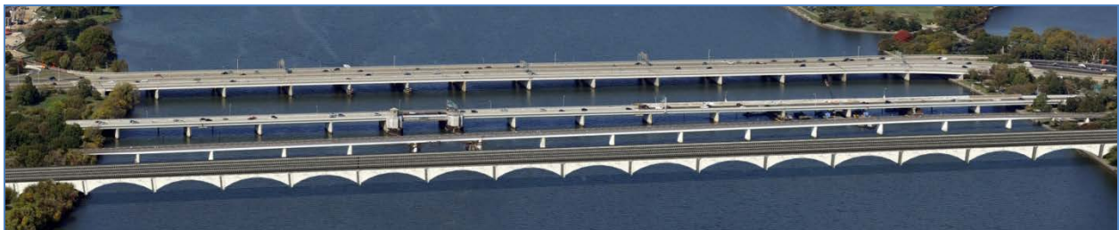
Figure 27 – Concrete Deck Arch Rendering of Long Bridge
