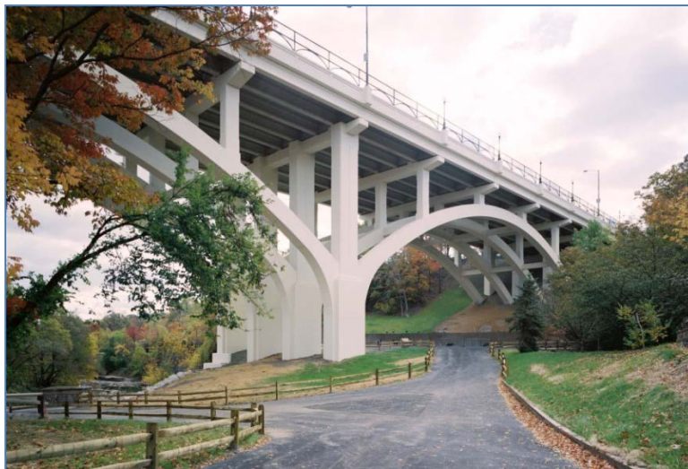
Figure 4 – Concrete Deck Arch Bridge
