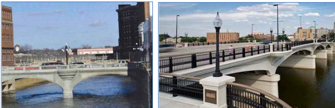
Figure 28 – Example of Precast Arch Facade Elements with Standard Girder Construction
