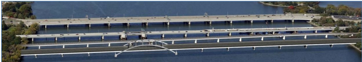
Figure 15 – Steel through Arch Rendering of Long Bridge
