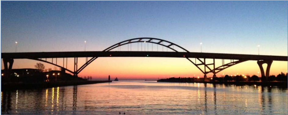
Figure 2 – Steel through Arch Bridge
