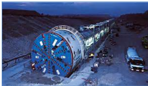
Figure 38 - Tunnel Boring Machine
