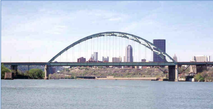
Figure 1 – Steel Tied Arch Bridge
