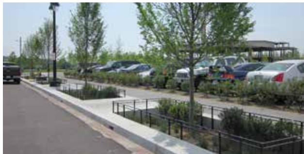
BIORETENTION PLANTER ADJACENT TO ROADWAY
