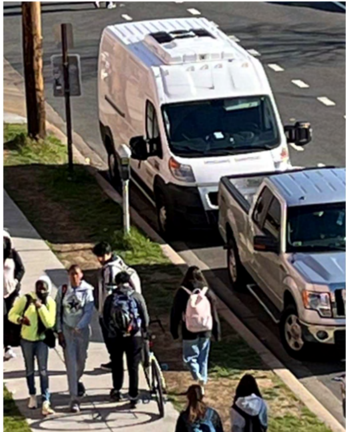
Six-foot sidewalk along 40th Street with wearing in the 5.5-foot grass section
