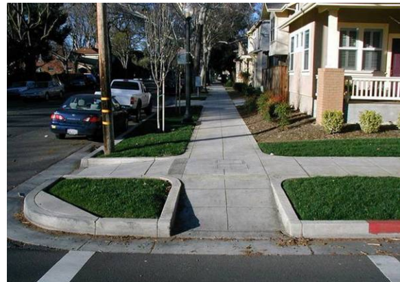
Figure 5 – Preferred sidewalk and ramp alignment at crosswalks – it is preferable to not provide a side flare adjacent to vegetated buffers.
