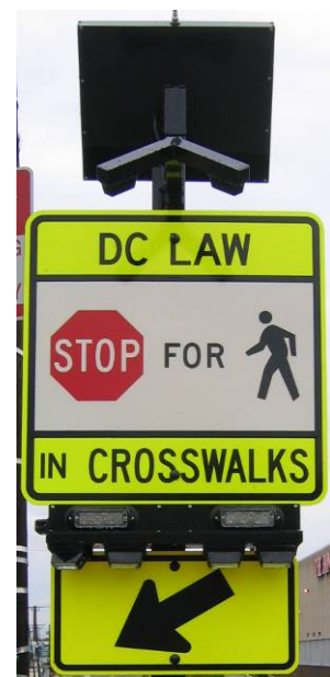
Figure 6 – Rapid Flashing Beacon with Side of Street Pedestrian Crosswalk Sign on Brentwood Road in Northeast DC
