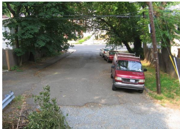
Figure 9 -W Place Alley looking towards 37 th Street
