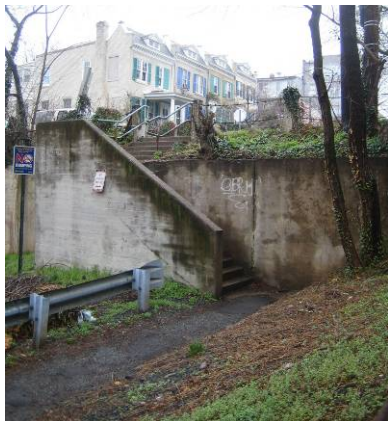
Figure 10 - Staircase view from W Place Alley
