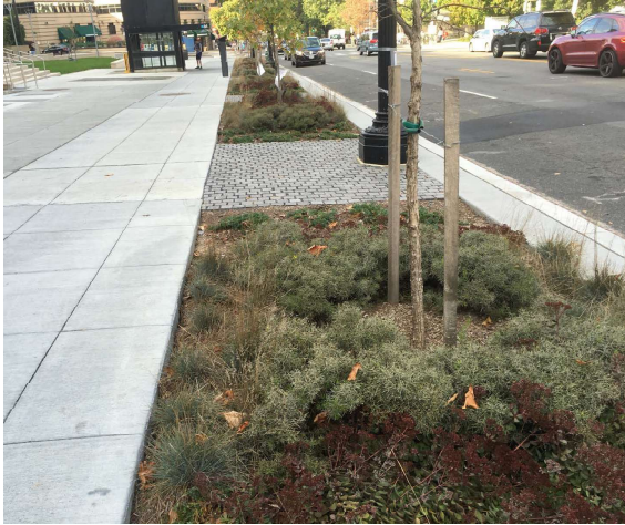
Step out zone: concrete pavers, 18 inches Tree pit: Min 6x10 ft; continuous preferred
