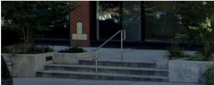
Stairs, ramps, walls: cast-in-place concrete Handrails: Stainless steel finish for building amenity zone
