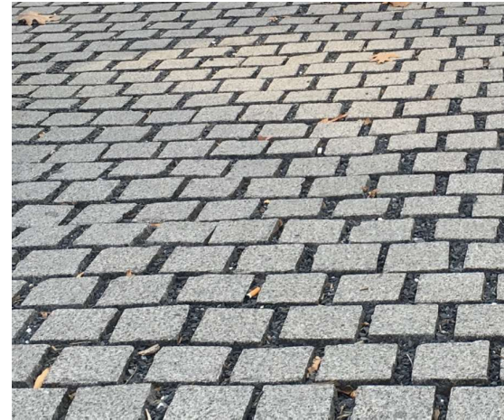
Pedestrian crossover: 4"x4"x4" pavers, Min. 6 ft wide
