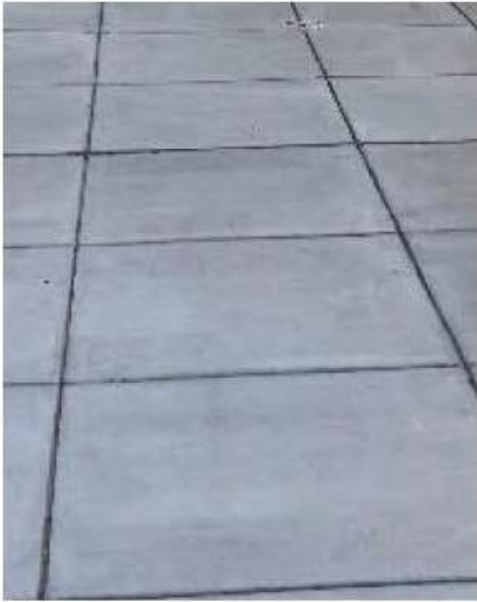
Scored Concrete Paving
