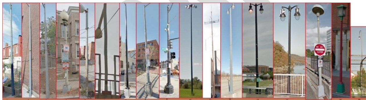
Types of DDOT Streetlight Poles in DC
