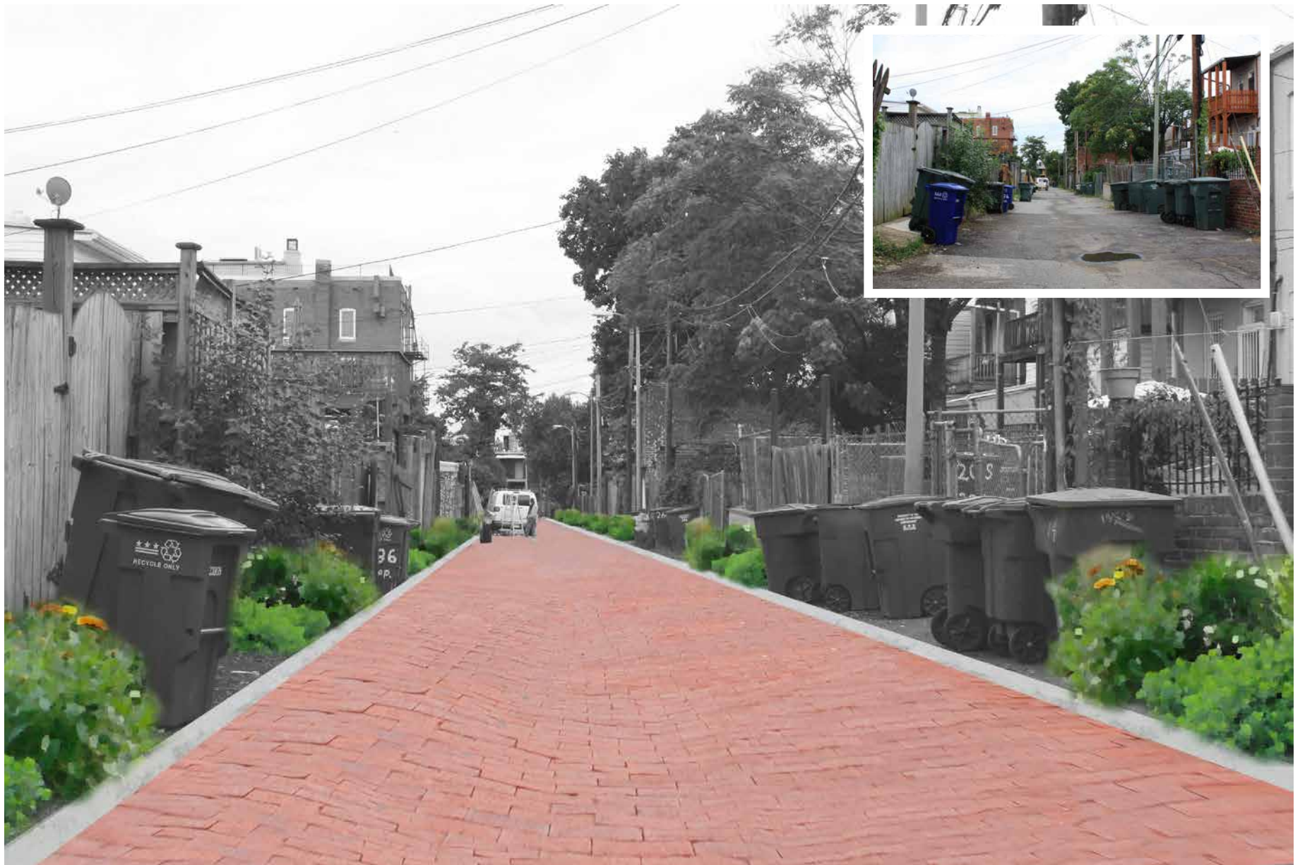
Figure 9-8 Green Alley Using Permeable Pavers
