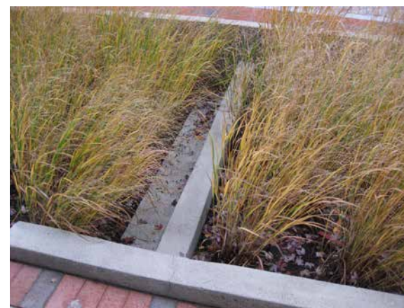
A check dam inside a tree box bioretention planter slows down the flow of water and encourages infiltration.
