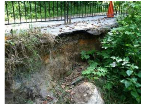
Slope Failure
