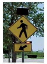
in a wig-wag "flickering" pattern at a rate of 70-80 periods per minute. The RRFB design differs from the flashing beacon by utilizing:
