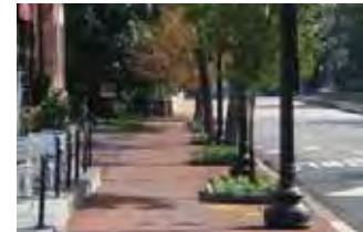
Properly Maintained Brick Sidewalk along M Street
