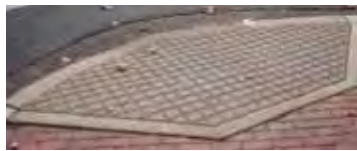
Brick-Patterned Curb Ramp
