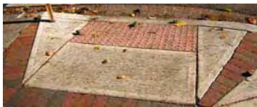
Curb Ramp with Detector
