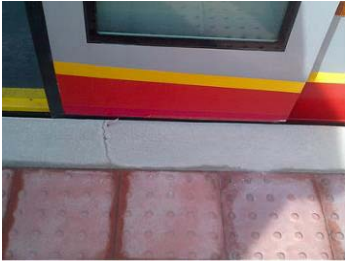
(Figure 4 – Inadequate clearance between platform edge and door opening.)
