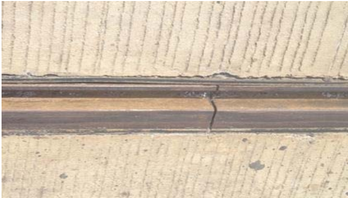
(Figure 1 – Rail break on mainline track)
