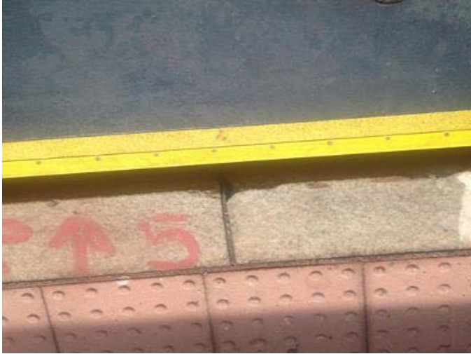
(Figure 8 – Platform edge showing the truncated domes and edge paving)
