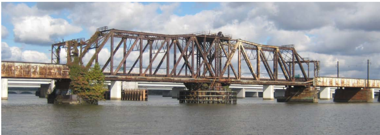
Long Bridge over Potomac River
