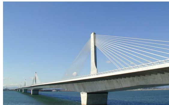
Example extradosed bridge
