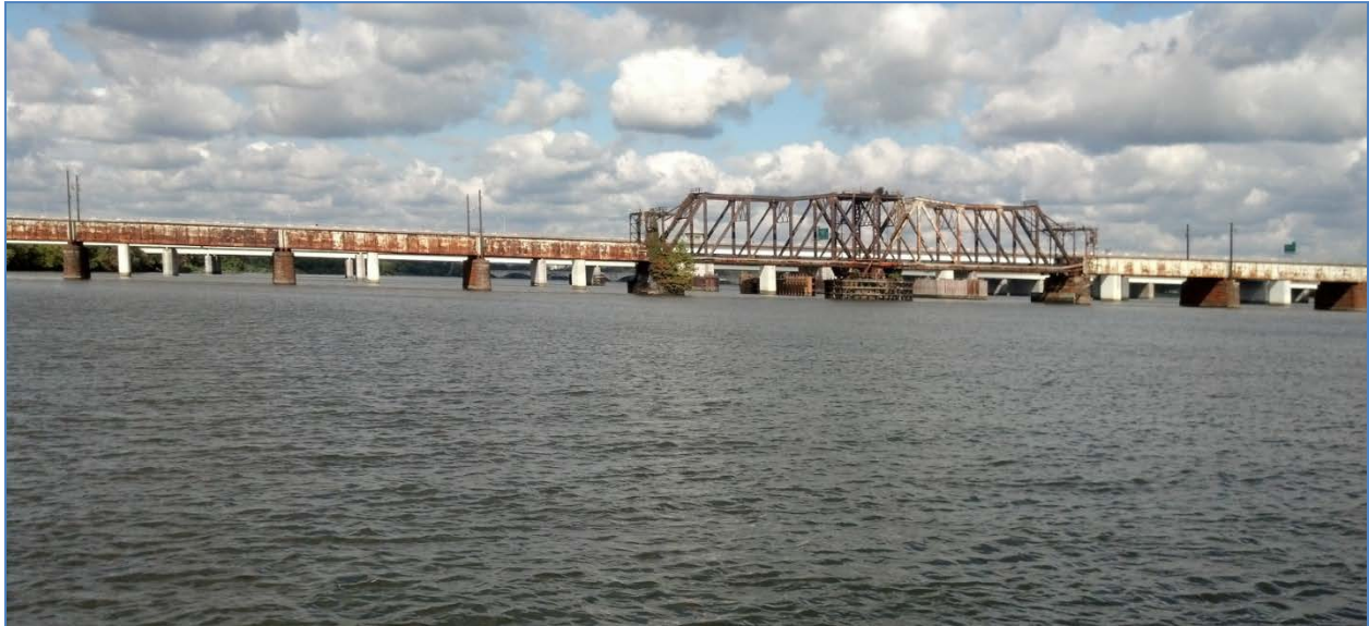
Figure 1 – Existing Through Girder and Truss Swing Spans
