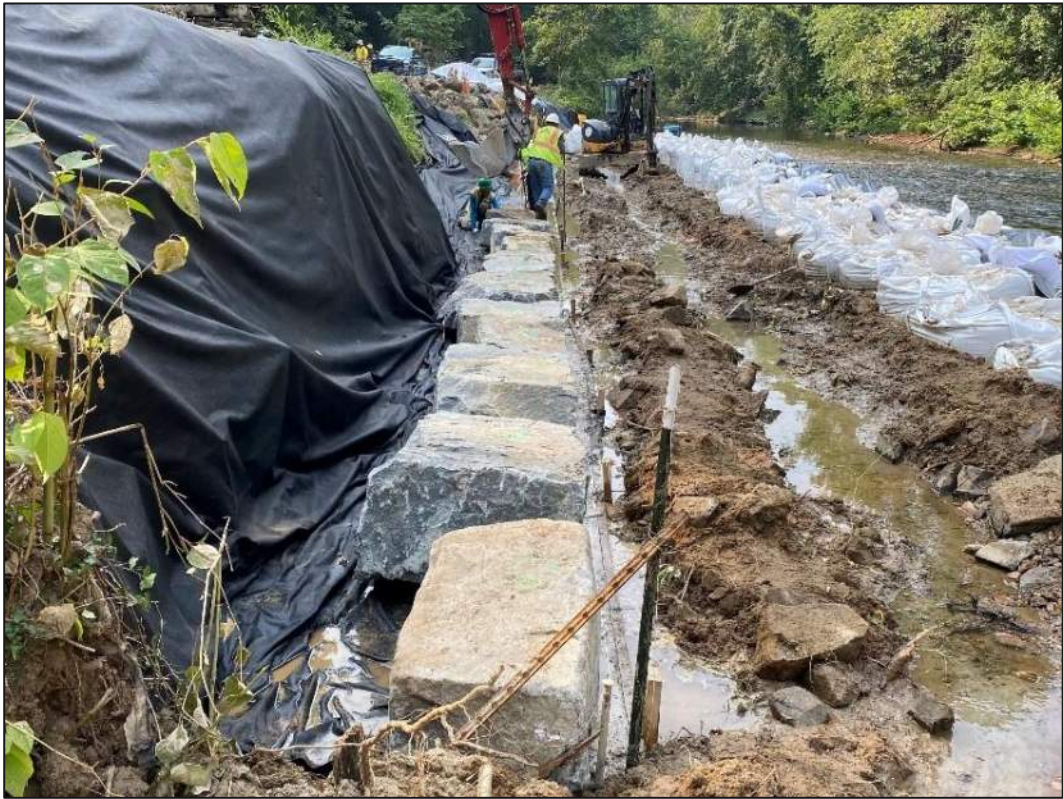
Restoration of eroded streambanks
