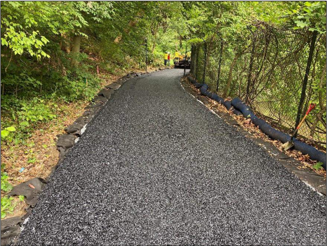
Permeable asphalt placement
