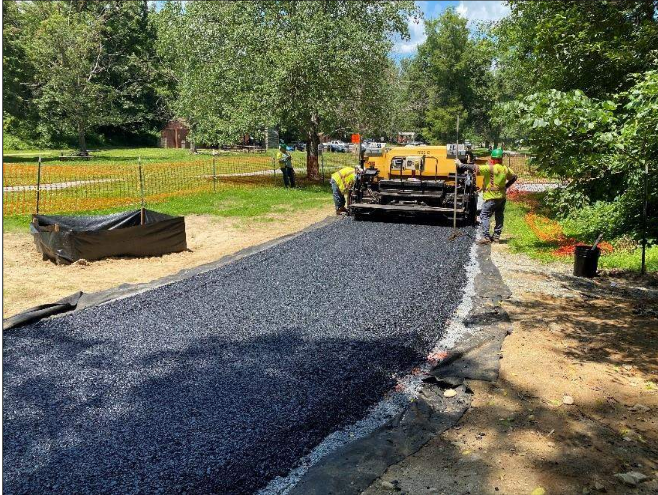
Placing new permeable pavement
