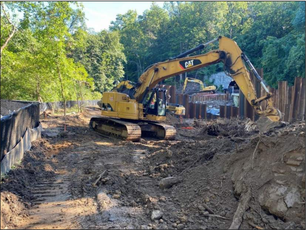
Excavation for bridge abutments
