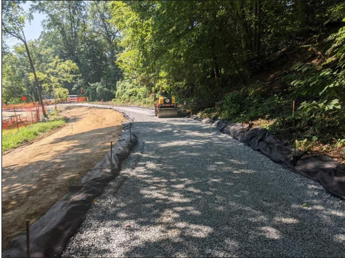
Preparing trail for permeable asphalt placement
