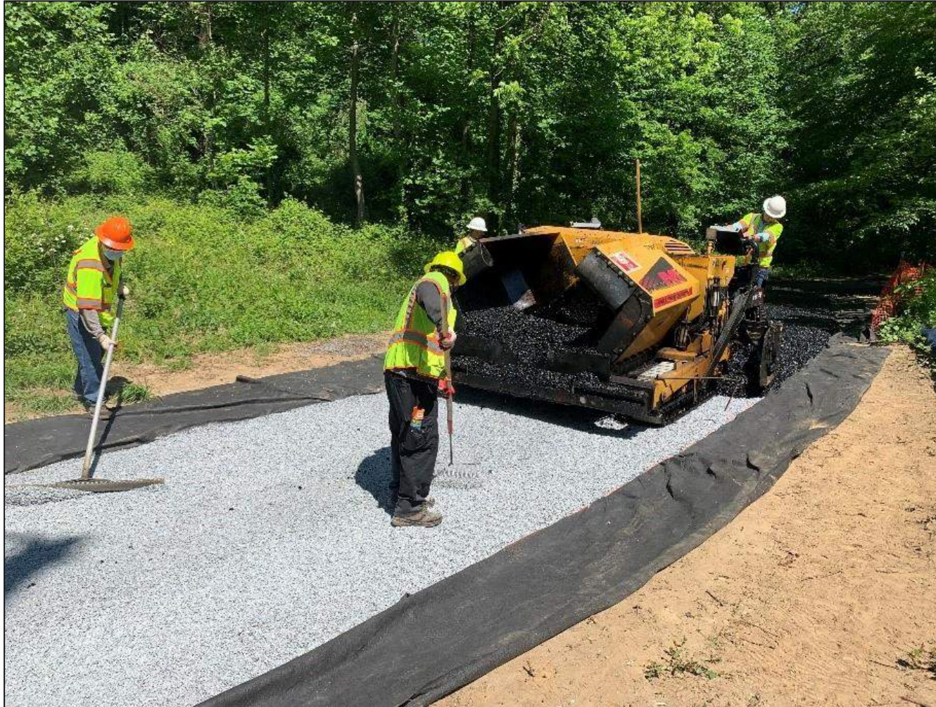
Permeable asphalt paving
